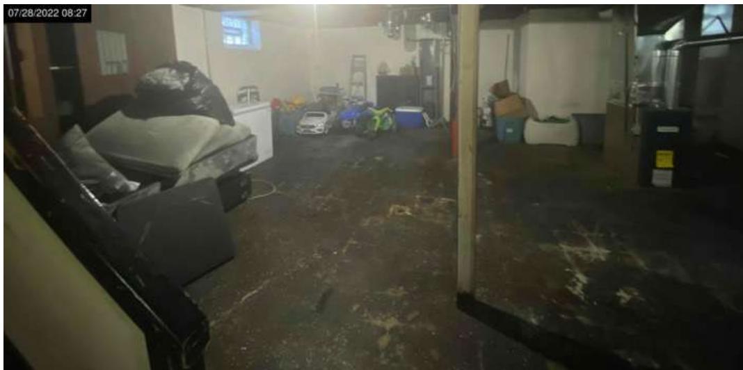
HVAC Interior Photos
